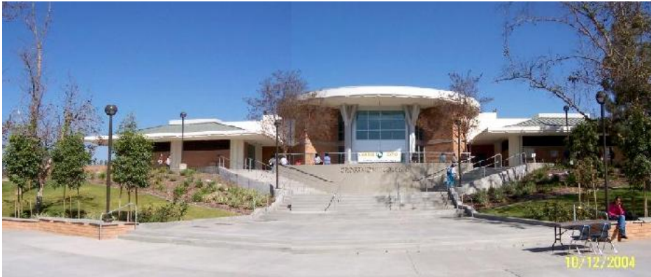
Dramatic overhaul of the LTRC facade and foyer (all photos by Bob Steinbach)
